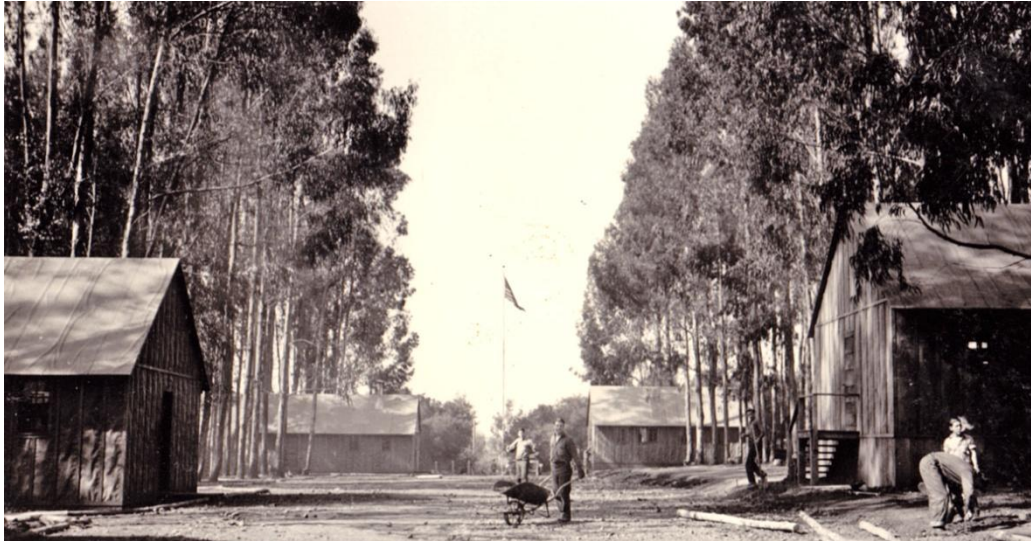
CCC Camp, under construction, February, 1934
